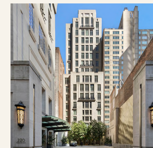
220 CENTRAL PARK SOUTH
